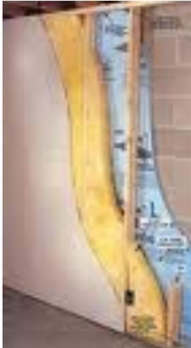
**Studded Basement Wall R-13 Cavity Insulation and R-5 foam backer**
