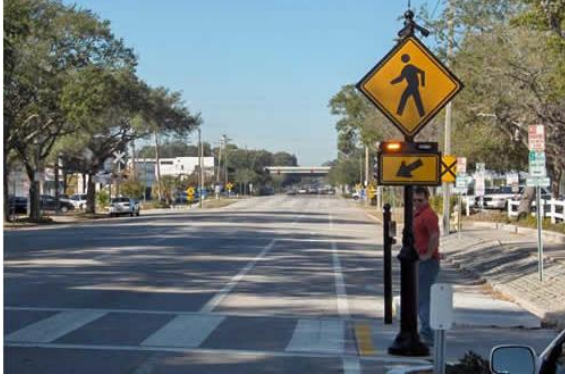
Left: Rectangular Rapid Flashing Beacon. Right: W11-15 and W16-7P signs.
